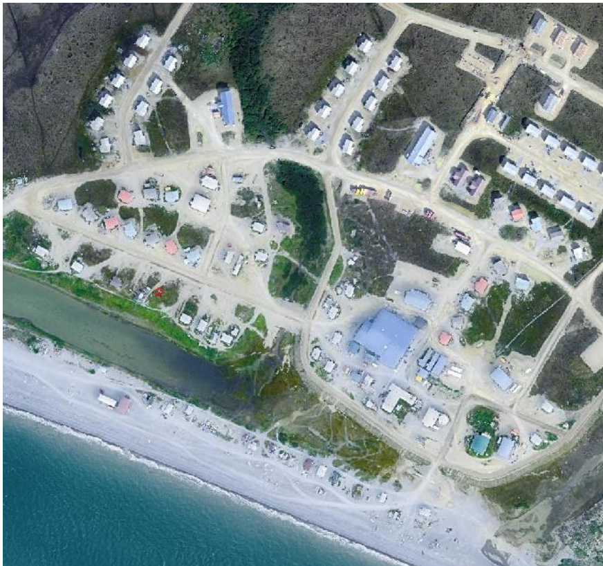
Examples of horizontal misfit assessment using village data, Brevig in this case. These images are from the coastal delivery. Flicker with the next page to see the village delivery. A 1-2 pixel offset was common.
